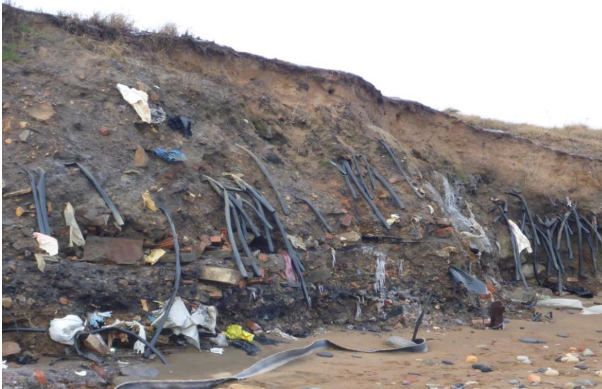
Figure 19 Landfill eroding from colliery spoil cliffs along open coastline north of the River Lyne
