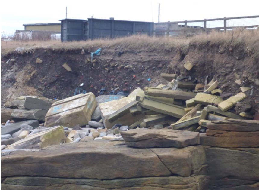
Figure 22 Foreshore littered with concrete rubble, with bricks, concrete and plastic eroding from Made Ground Cliffs along coastline of site Reference 4
