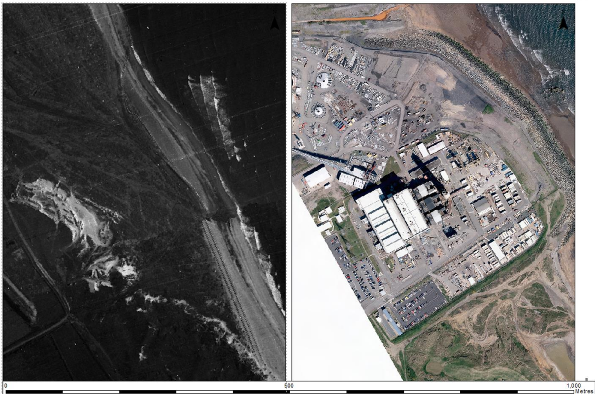
Figure 30 Site of Lynemouth Power Station in 1940 (left) and 2017 (right)
